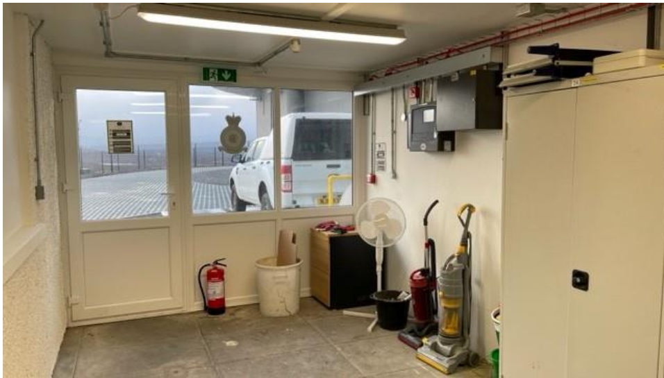
Fig 2 Fire Panel location
