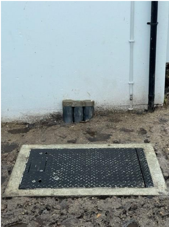
Fig 1 Lightning band and ducting
