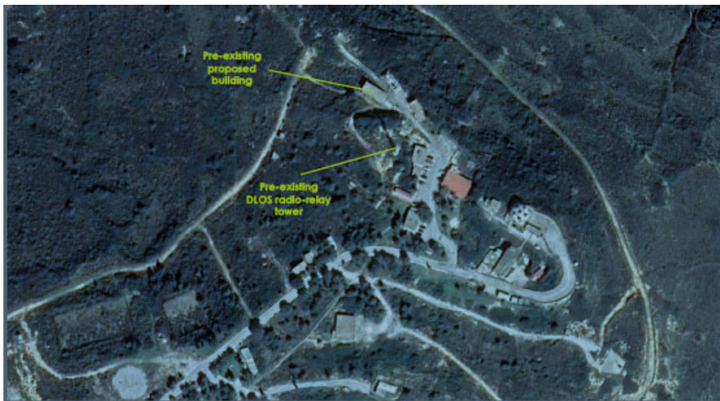
Figure 6: New UHF Site 7th Air Force Radar Station (Skyros Island)
