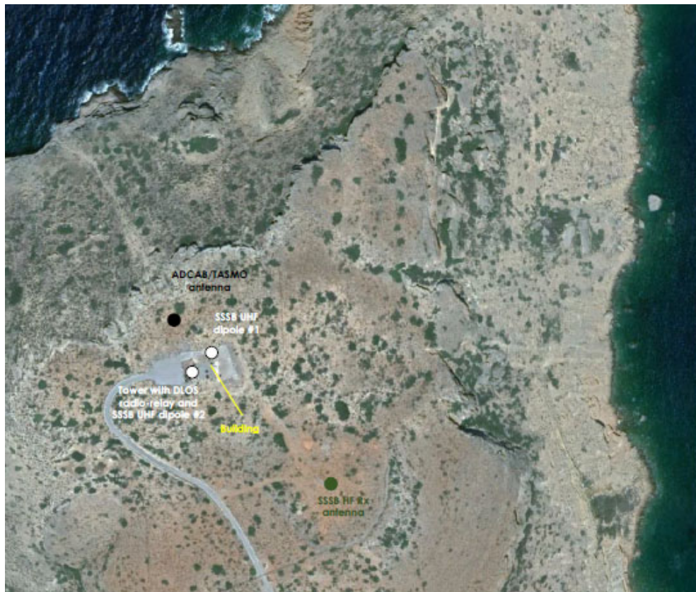
Figure 8: HF-TX/UHF site Cape Mavros (Crete Island) Current Site Configuration
