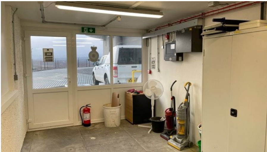
Fig 2 Fire Panel location
