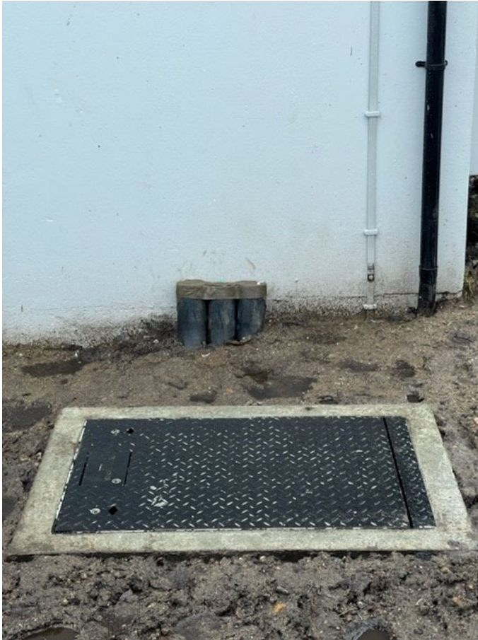
Fig 1 Lightning band and ducting
