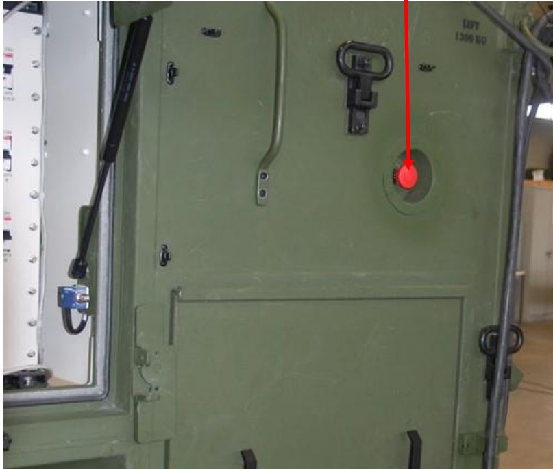
TSGT Container Left Side Emergency Power Off
