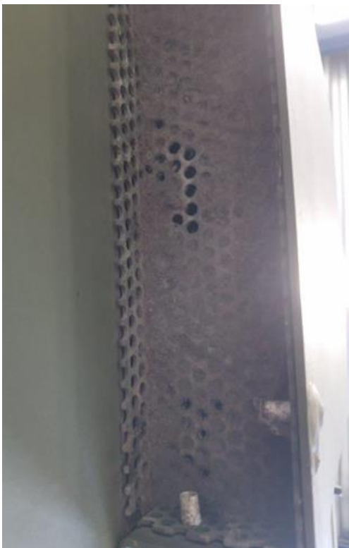
Figure 3.2.2.2-1 Dirty GPFU Air Intake
