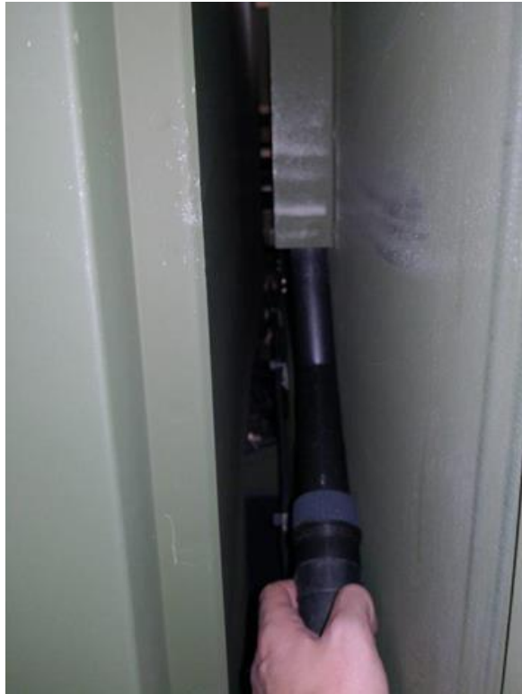
Figure 3.2.2.2-3 Cleaning GPFU Air Intake on Mounted Container
