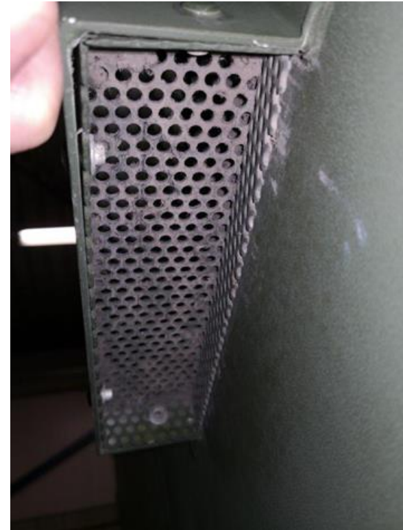
Figure 3.2.2.2-4 GPFU Air Intake After Cleaning
