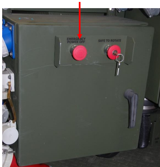
T-1 Extension Trailer Power ETB Emergency Power Off Button
