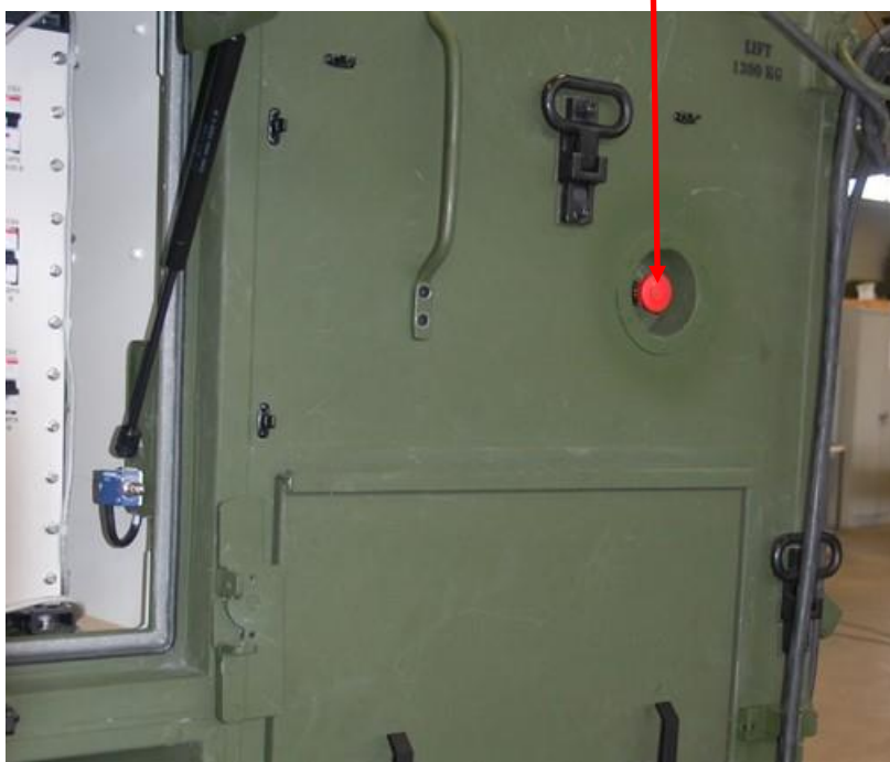
TSGT Container Left Side Emergency Power Off
