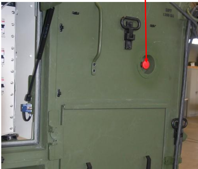
TSGT Container Left Side Emergency Power Off
