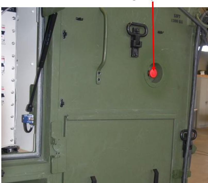
TSGT Container Left Side Emergency Power Off
